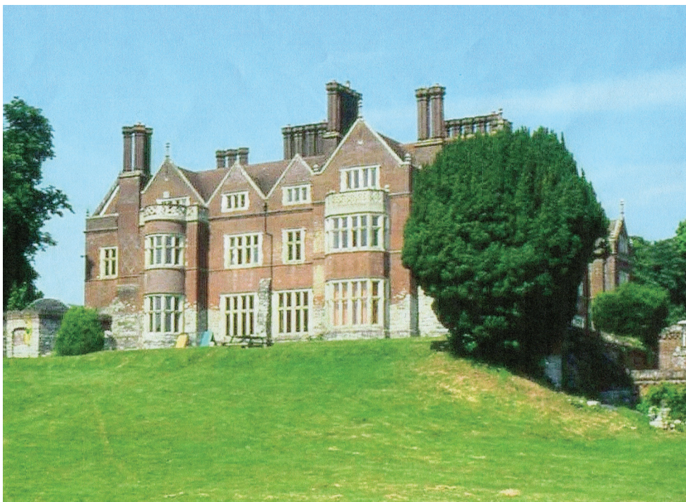
Fig. 3 The 1878 replacement St Alban's Court
