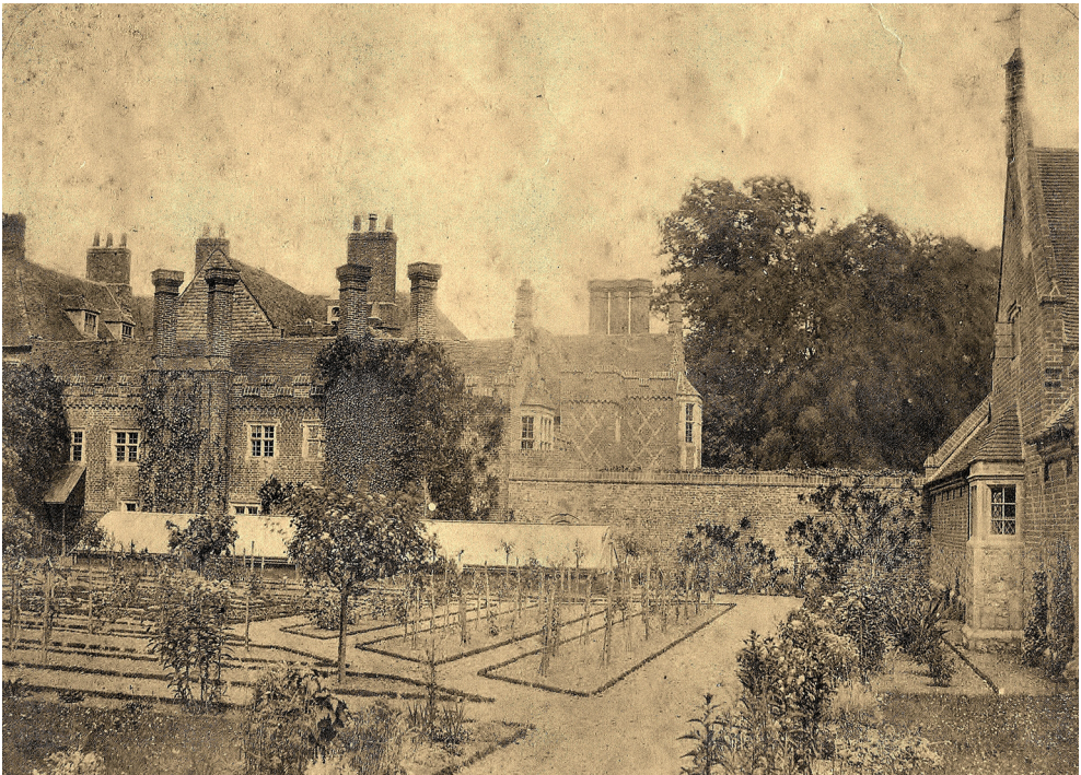
Fig. 6 Old St Alban's Court: south-west (flower garden) elevation; photo 1869.
